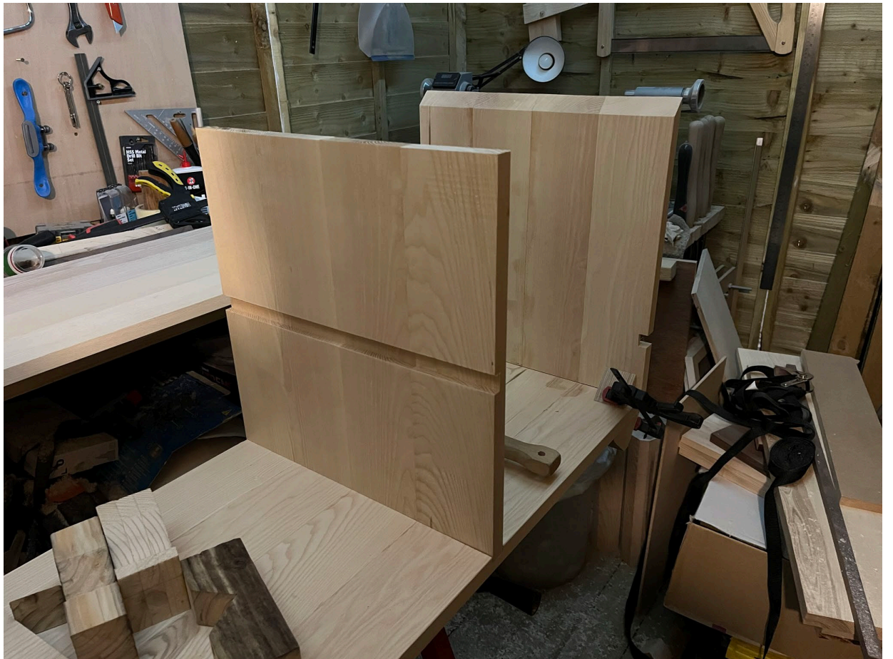
Hand planing corners and dry fitting
