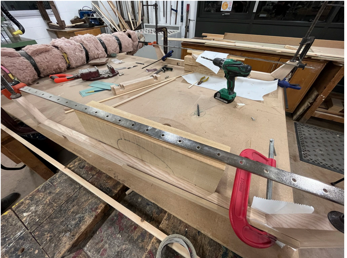
Gluing the feet
