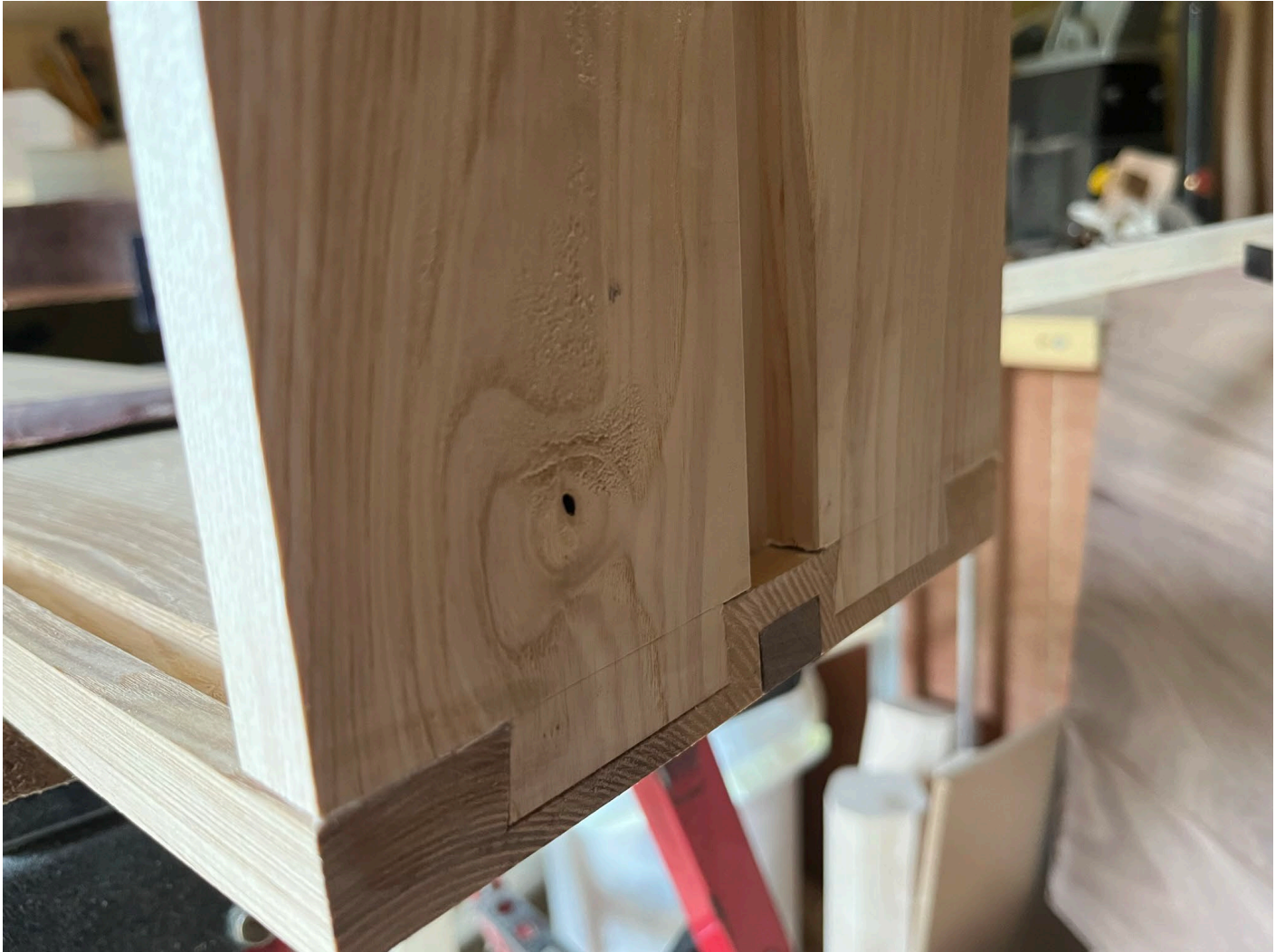
Half-blind dovetail joint
